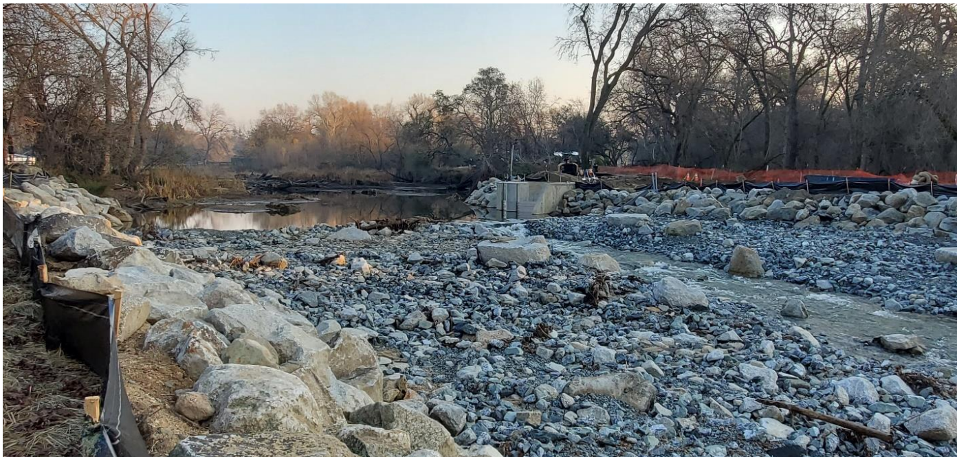
In this early-December photo, the old dam has been removed and replaced with a new "nature-like" system. The concrete walls of the canal intake can be seen in the distance just to the right of center. (Friends of Auburn Ravine Photo.)
